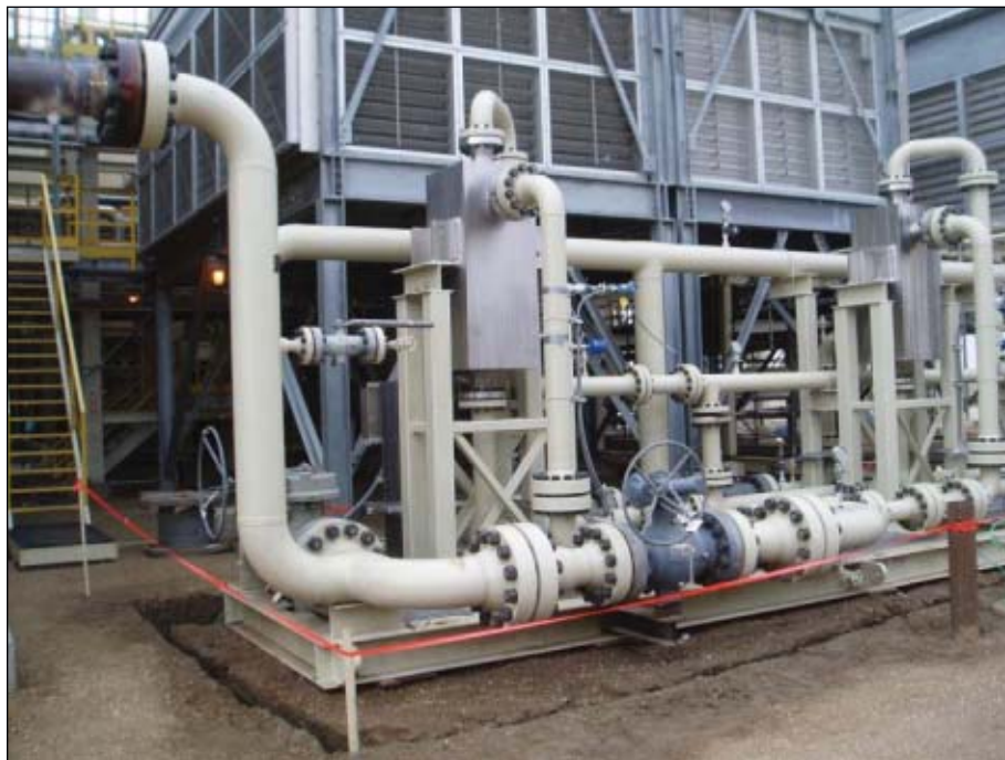
To minimize size constraints in the facility, the project installed compact printed-circuit heat exchangers (Fig. 4).
