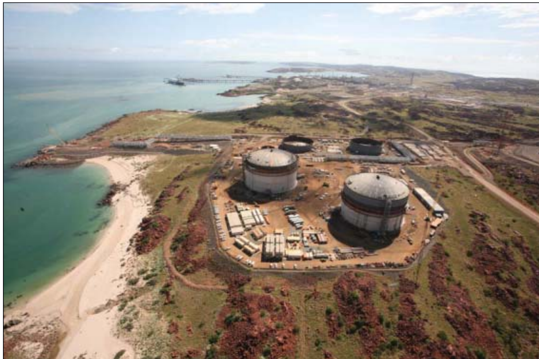
For Woodside Petroleum Ltd.'s Pluto LNG Project, CB&I is supplying two 120,000-cu m LNG storage tanks as well as additional condensate tanks. The Pluto LNG liquefaction facility, built on the Burrup Peninsula in Western Australia, is expected to produce 4.3 million tonnes/year of LNG. Photo from CB&I.
